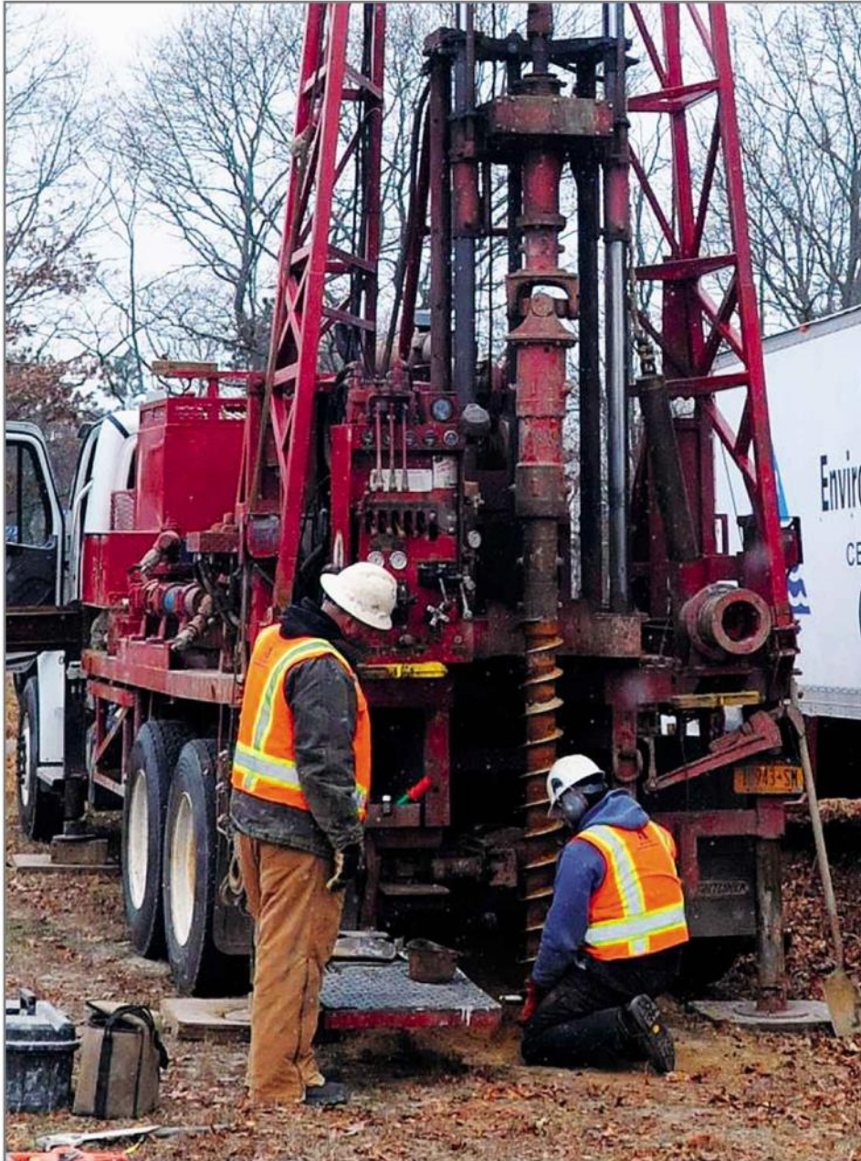
A well is dug at Roberto Clemente Park in Brentwood last month. The county will sink its own monitoring wells at the park and at other sites. ■ Photos, updates: newsday.com/toxicdumping
